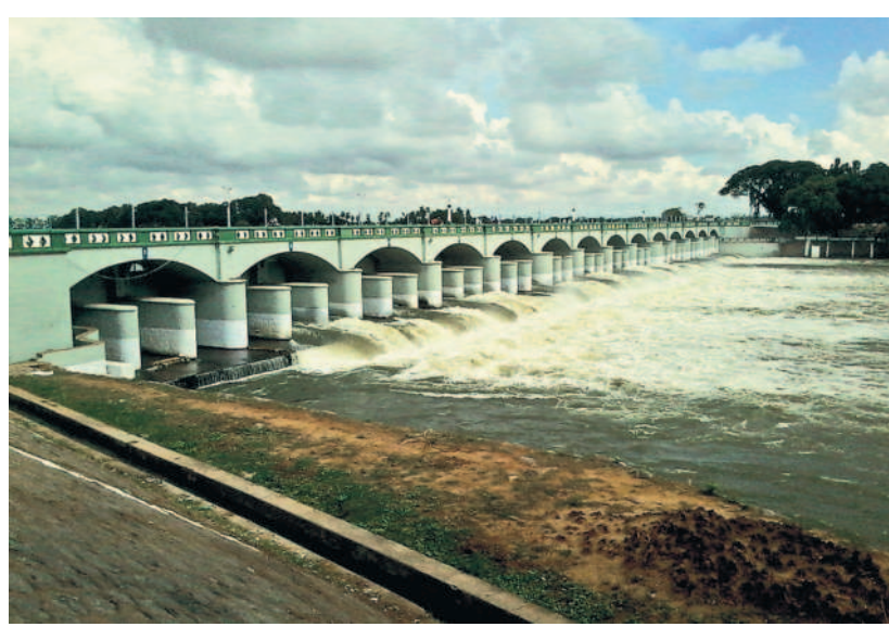
The Kallanai Dam across the Kaveri, built by Karikala Cholan and still operational today, is also known as the Grand Anicut. LOKESH RAMACHANDRA, WIKIMEDIA COMMONS
